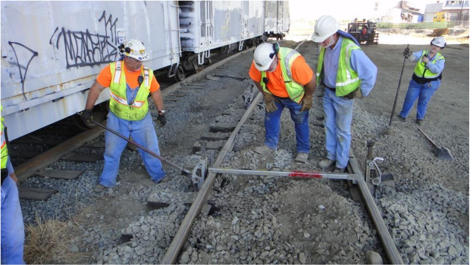
Heather supervises Frank and Mike M. as they check the level while Mike F. jacks the north rail even with the south
