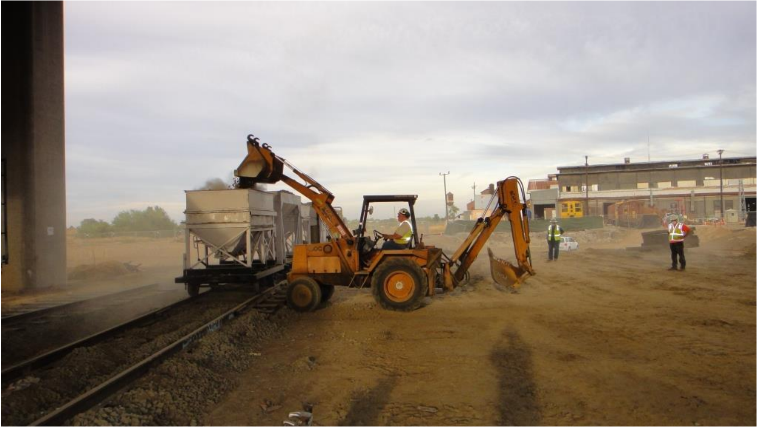
Frank W. in the back-hoe loads rock in a hopper as Frank S. and Fred stand by to spread it about
