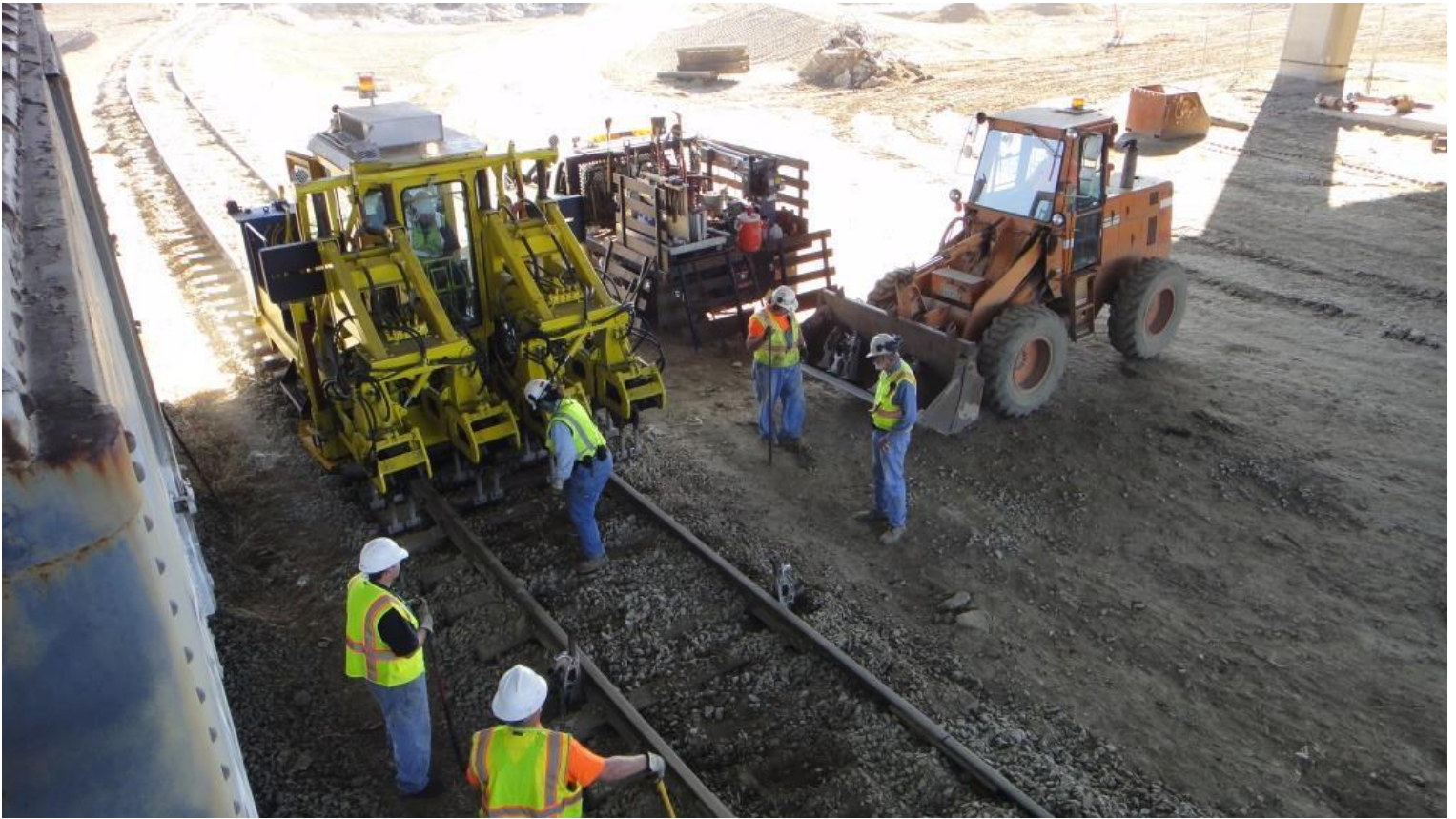
Heather guides Harry in the tamper while Randy, Scott, Mike and Alan pull jacks and put in the bucket of the loader which Frank is running
