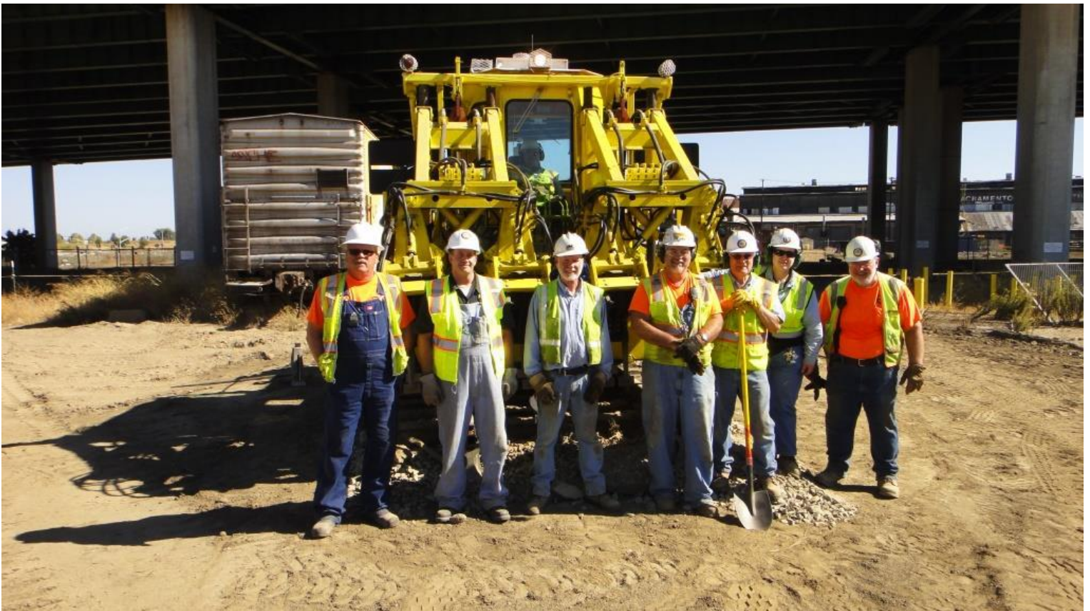
Saturday's fantastic Team that completed the building of the new Rail Yards Storage Track: Scott, Randy, Mikes M., F., and W., Heather, Frank, and Harry in the tamper
