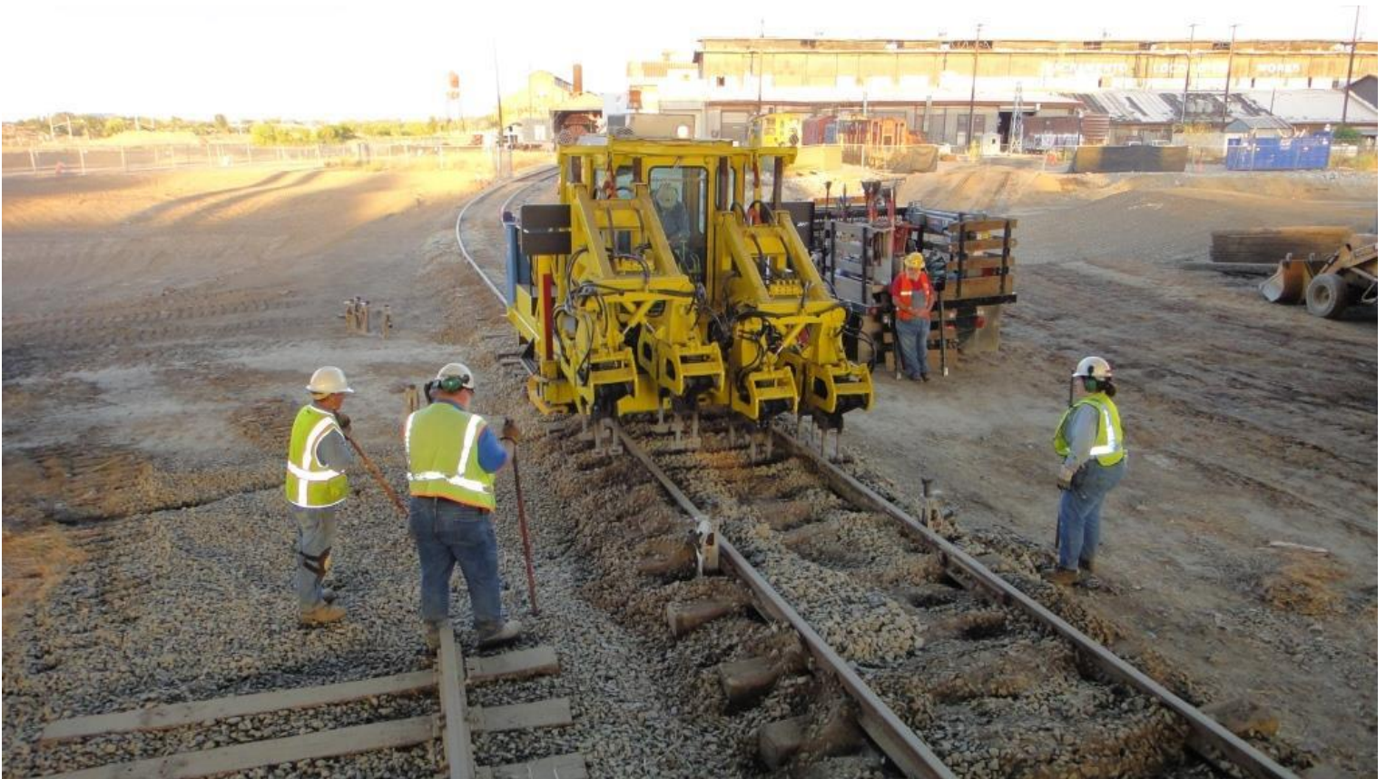
Alan tamps the track while Mike T., Frank, Pat, and Heather pull jacks
