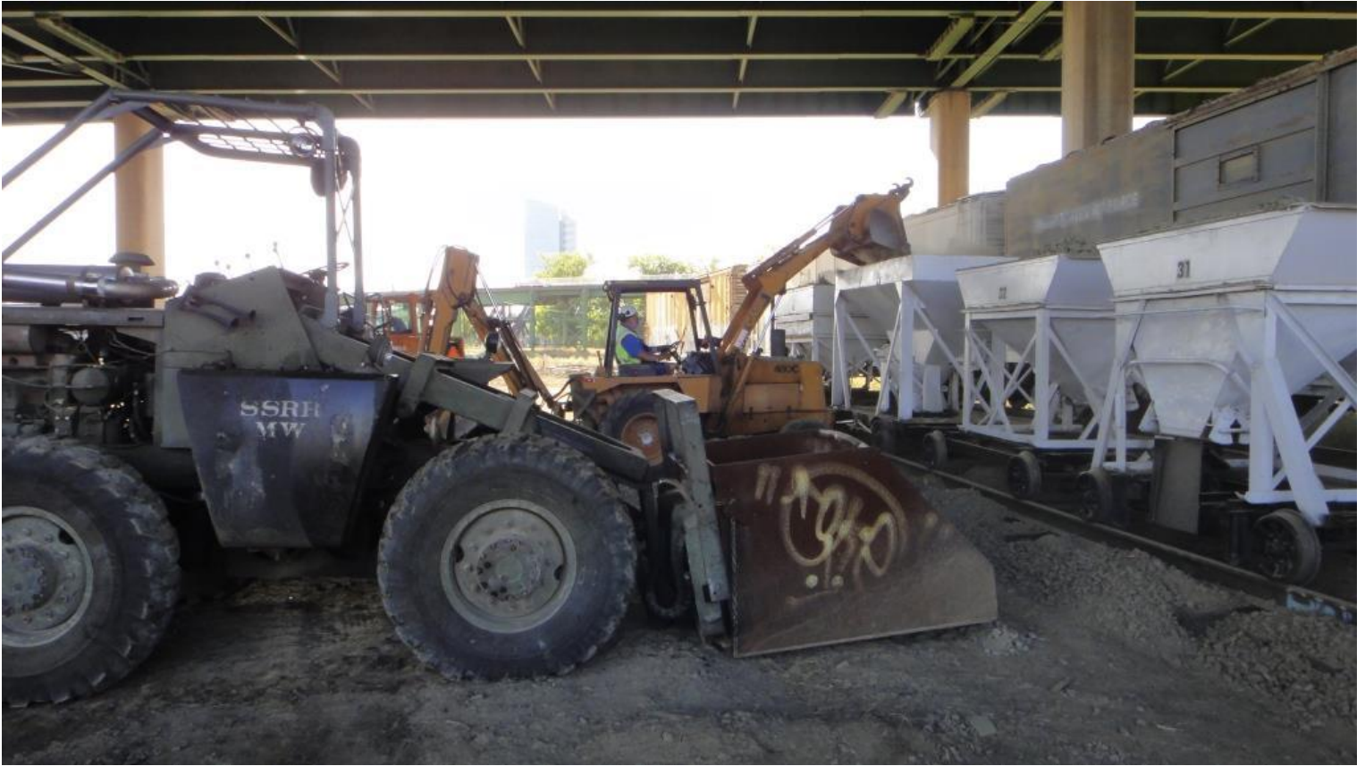
Frank loads rock into the center-dump hopper
