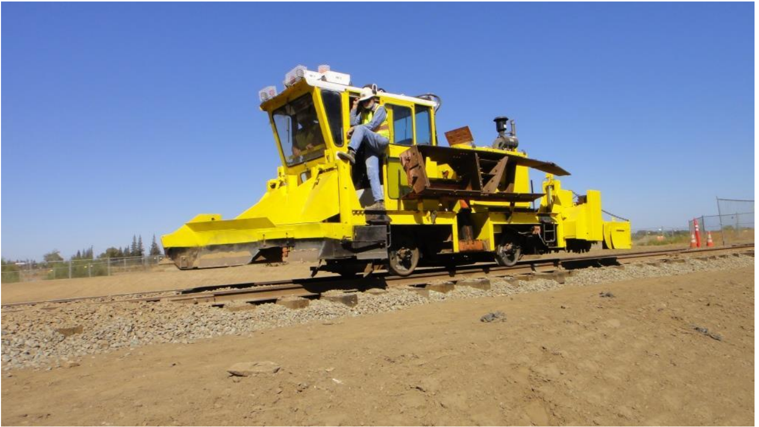
Bring in the Sea Tiger ! The final step, the ballast regulator plows the rock between the rails
