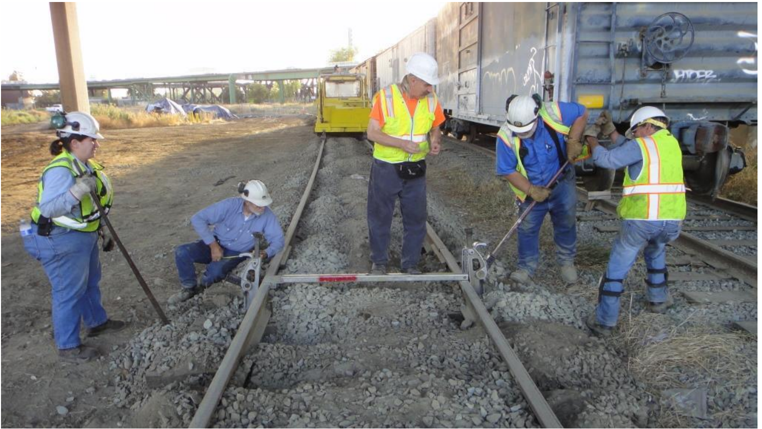
After Heather jacked-up the south rail, Frank and Mike T. team-up to jack the north rail level while Alan and Fred spot the level
