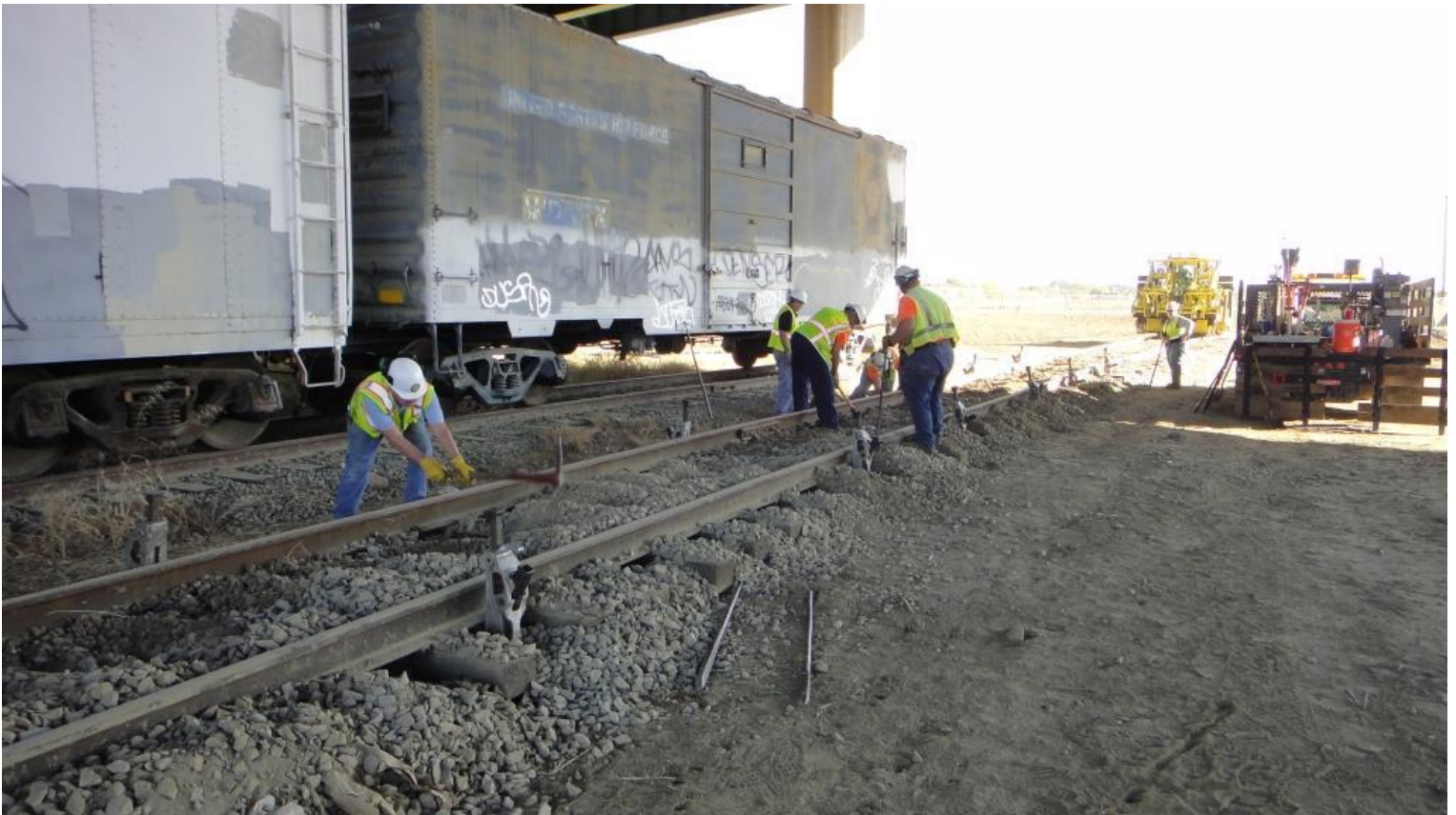
Mike W., Randy, Scott, Frank, and Mike F. set jacks to line and level the track
