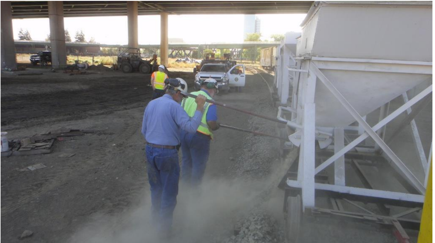
Alan and Frank disgorge rock from the side-dump hopper
